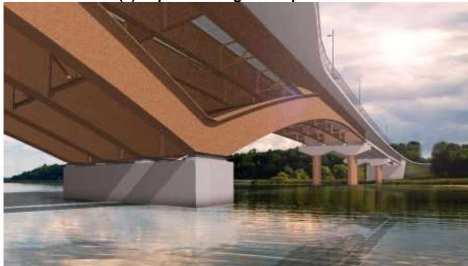
(b) Vertical Navigation Span Piers
