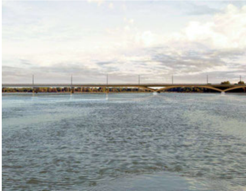
Figure 1-8: View of Bridge from Navigation Channel from 200 m
