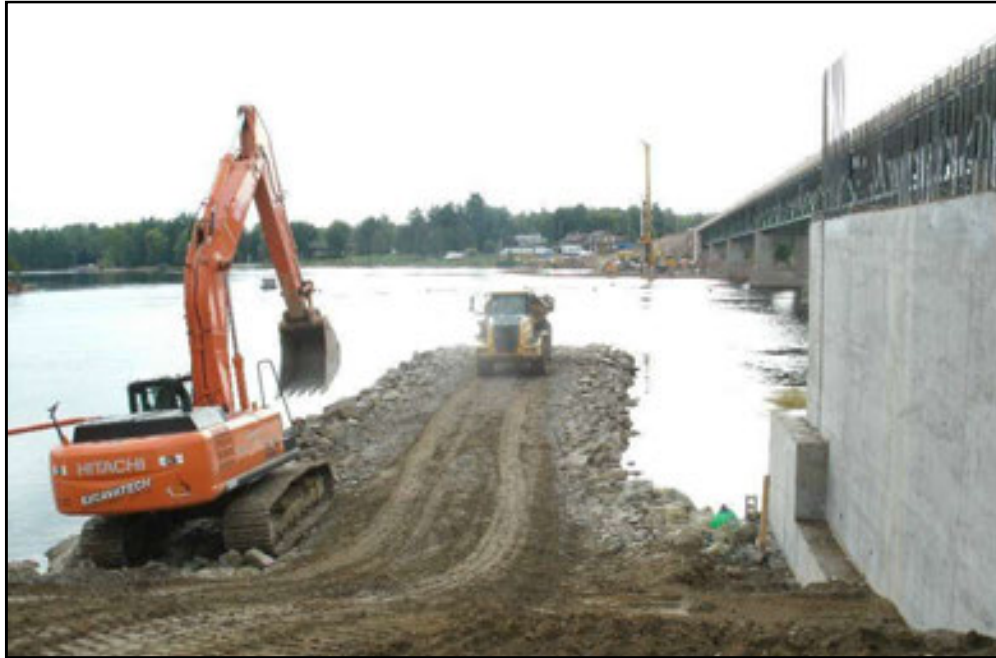
Figure 2-2: Temporary Earth Berm
