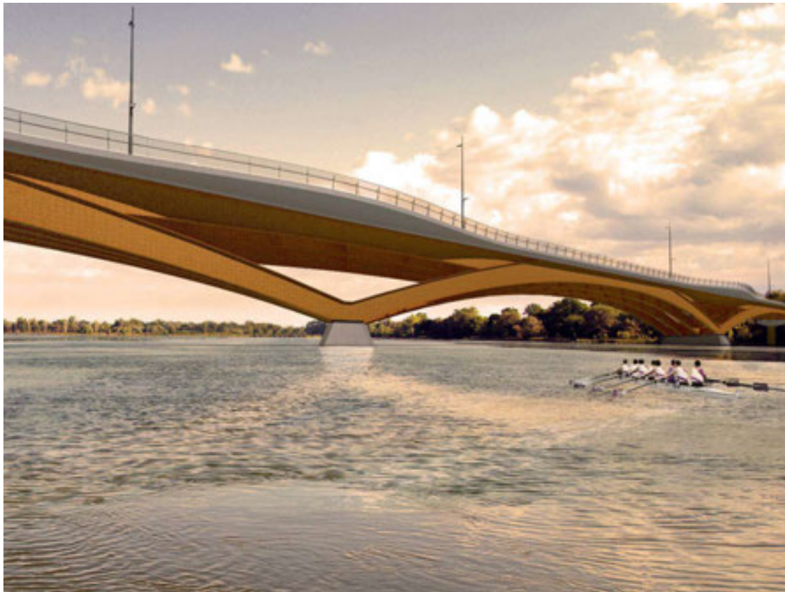
a) View Near the Navigation Channel Span
