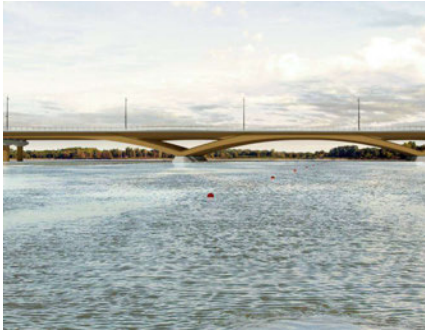
Figure 1-9: View of Bridge from Navigation Channel from 100 m
