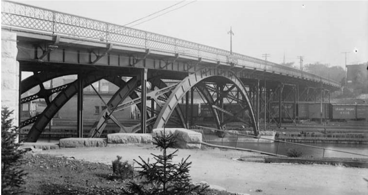
Figure 1-15: Historic Laurier Bridge over the Rideau Canal
