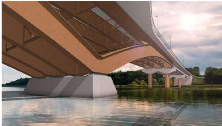
(a) Tapered Navigation Span Piers
