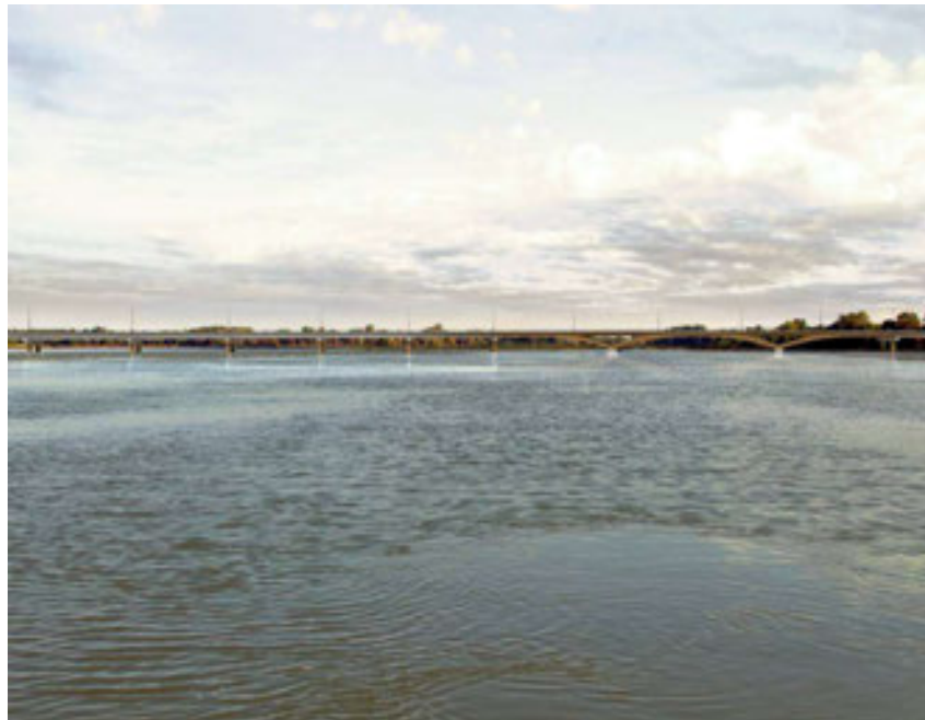
Figure 1-7: View of Bridge from Navigation Channel from 300 m
