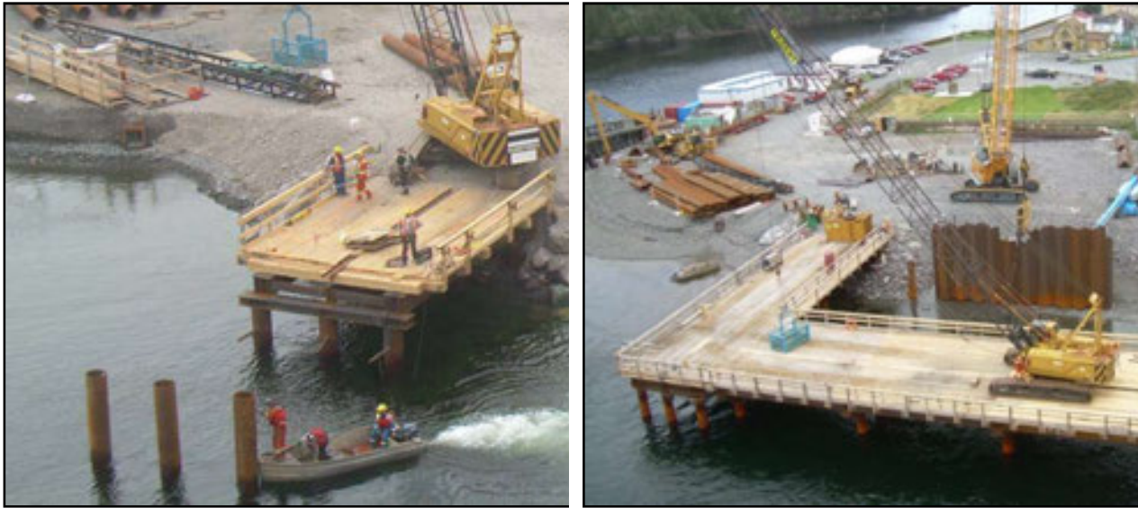
Figure 2-3: Trestle or Temporary Work Bridge
